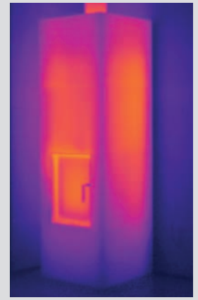
12 hour after heating Average surface temperature 45 °C
